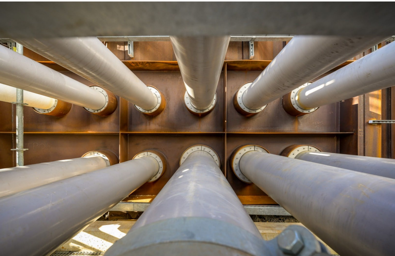
** Figure 2. Off-center Seals installed in steel wall
