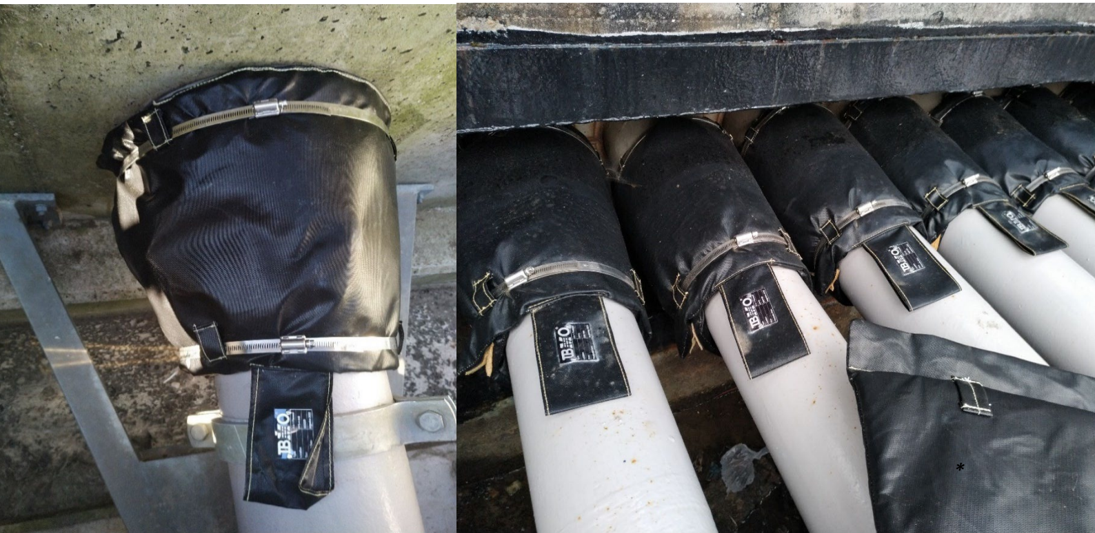
Figure 4. 3 in 1 Wrap Seals bund wall penetrations
