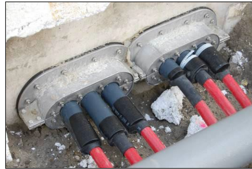
Situation after installation of front flange
