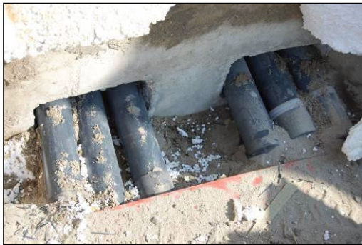
Position for installing the front flange
